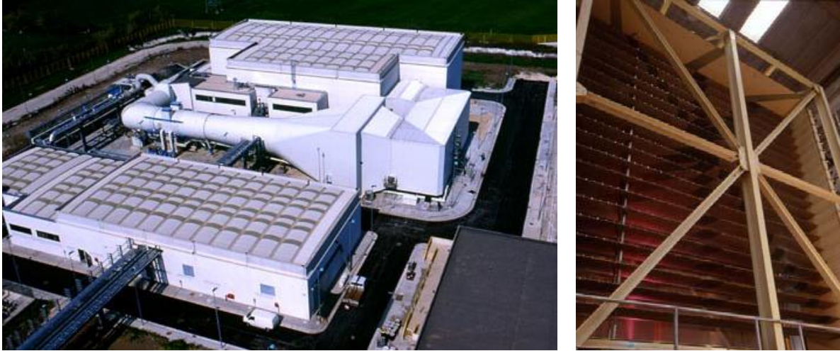
Fig. 1: General view of the Icing Wind Tunnel (IWT) and close-up of the spray bar system
