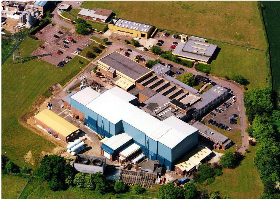
Aerial View of the ARA Transonic Wind Tunnel
